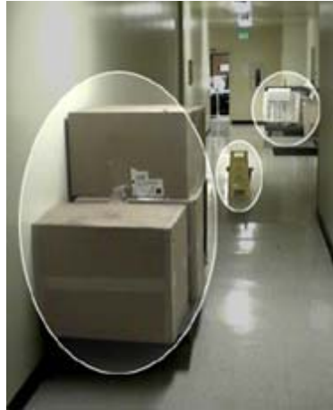
Obstructed exit route
