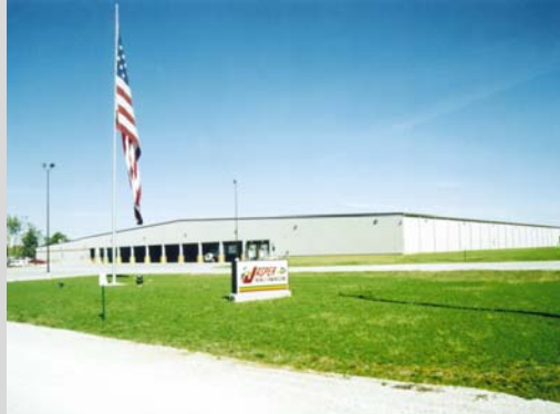
1999 - Completion of core processing and distribution center in Crawford County
