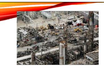
At approximately 1:20 p.m. on March 23, 2005, a series of explosions occurred at the BP Texas City refinery during the restarting of a hydrocarbon isomerization unit. Fifteen workers were killed and 180 others were injured. Many of the victims were in or around work trailers located near an atmospheric vent stack. The explosions occurred when a distillation tower flooded with hydrocarbons and was overpressurized, causing a geyser-like release from the vent stack.
